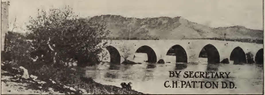
The Roman Bridge at Missis
